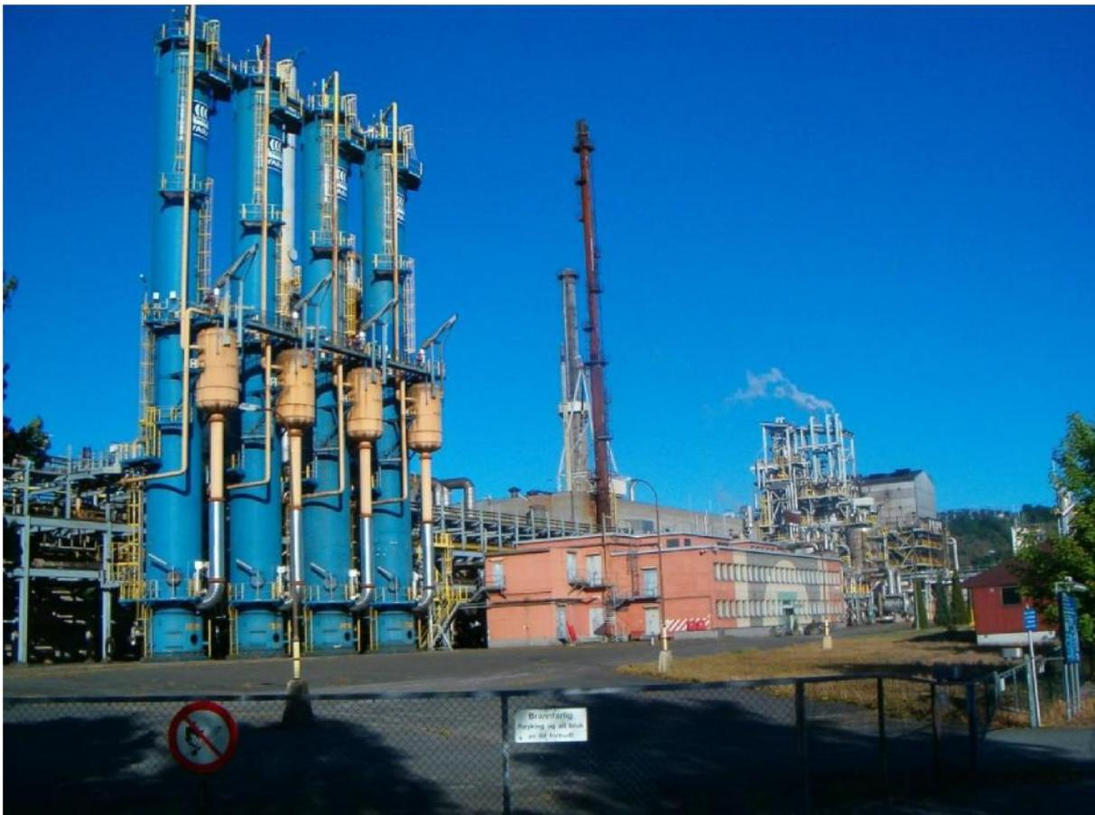
*Figure 5.4.1 Ammonia plant N2 in Porsgrunn. In the four water wash towers in the foreground, CO<sub>2</sub> is removed from the process gas.*
