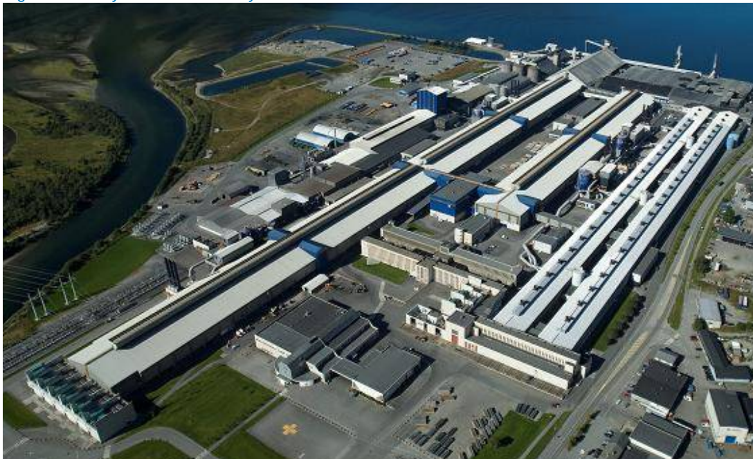
Figure 4.1: Hydro Sunndal facility
